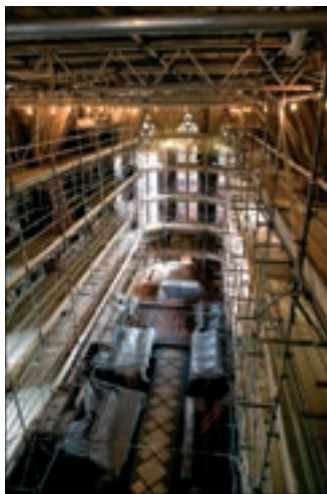
The Chapel interior under scaffolding, 2007
