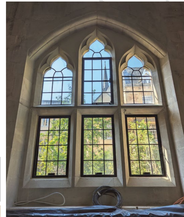
THE FULL HEIGHT OF THE ANNEXE'S GOTHIC WINDOWS HAS BEEN REVEALED
