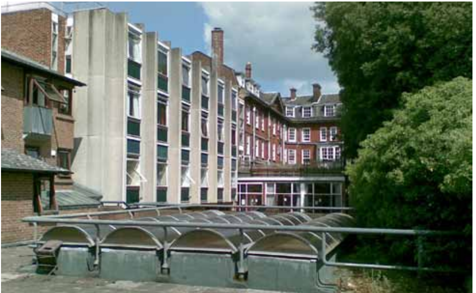
The inner courtyard as it currently looks
