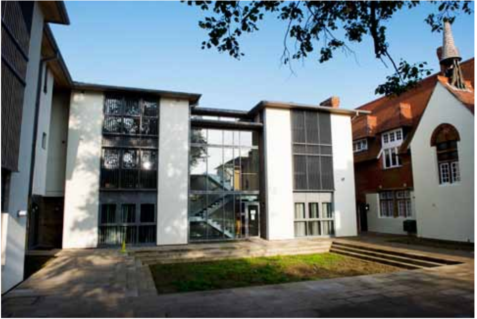
Two views of the impressive new accommodation built at the Exeter House site
