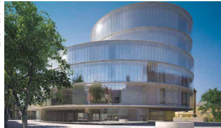
Southern side of the Blavatnik School of Government
