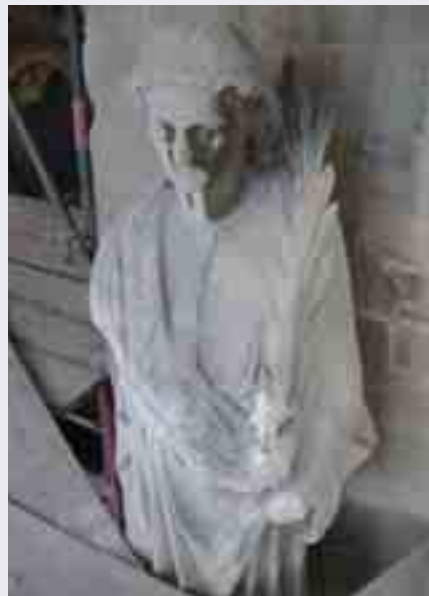
ABOVE: ST. ANDREW IS TAKEN TO THE MASON'S YARD. RIGHT: REPAIRING ST. ANDREW WOULD HAVE MEANT CUTTING OUT OVER 50% OF THE OLD STONE, SO IT WAS DECIDED PREFERABLE TO HAVE A NEW ONE CARVED. SCULPTOR CORIN JOHNSON MAKES A START AT JOSLIN'S YARD. BELOW: ST. JOHN, BEFORE AND AFTER
