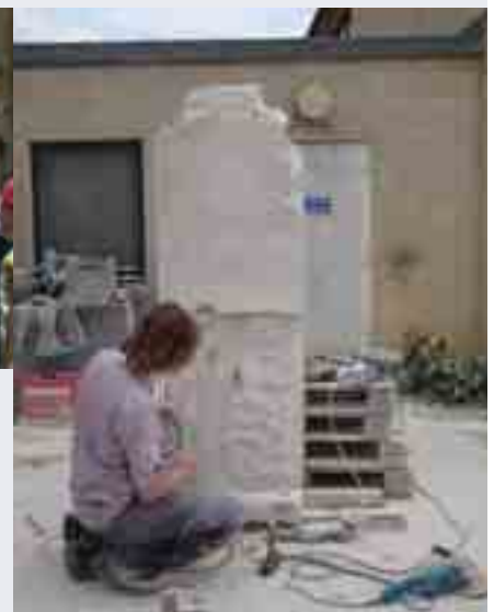
ABOVE: ST. ANDREW IS TAKEN TO THE MASON'S YARD. RIGHT: REPAIRING ST. ANDREW WOULD HAVE MEANT CUTTING OUT OVER 50% OF THE OLD STONE, SO IT WAS DECIDED PREFERABLE TO HAVE A NEW ONE CARVED. SCULPTOR CORIN JOHNSON MAKES A START AT JOSLIN'S YARD. BELOW: ST. JOHN, BEFORE AND AFTER
